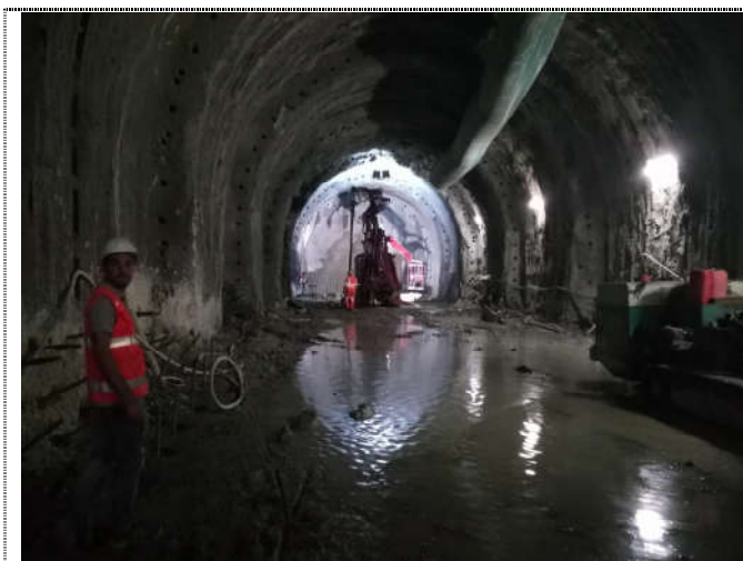
Figure 15. Final excavation phase
