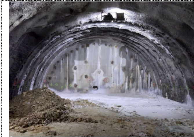
Figure 13. First phase excavation – jet grouting columns
