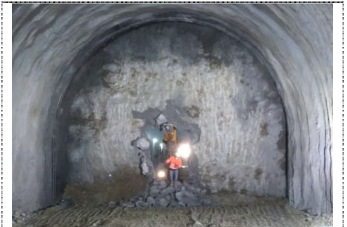
Figure 16. The excavation of tunnels is completed
