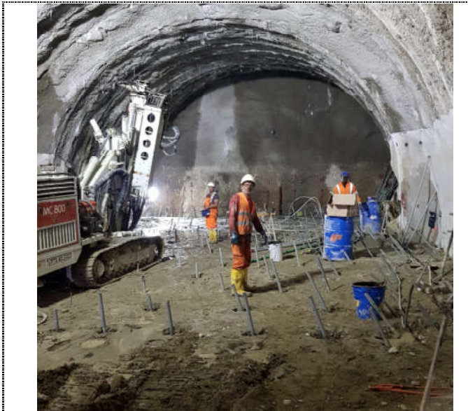
Figure 14. First phase excavation – subvertical grouting treatments
